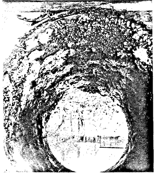
Fig. 4. The same main as shown in Fig. 3, Plate 1, before treatment in January 1950. The white patches in Fig. 3, Plate 1, are sponges
